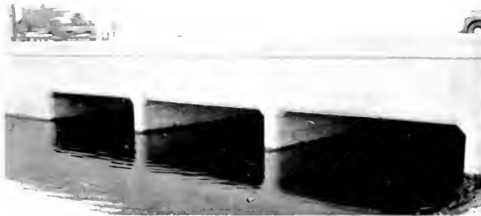
FIG. 19. Rounded-lip entrance to concrete box culvert
